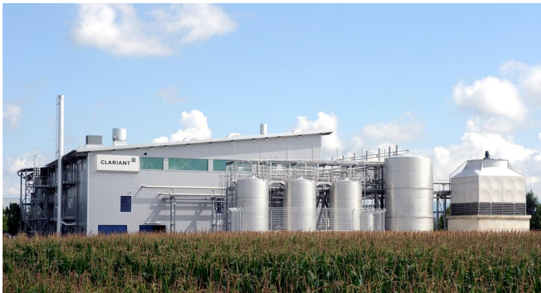
Extensive tests with Enviral's feedstock were conducted at Clariant's pre-commercial plant in Straubing, Germany. (Photo: Clariant)
